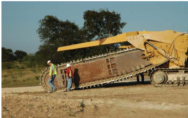
Trenching Machine Used in Biowall Construction
