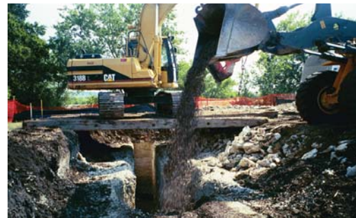
Media Backfilling of Biowall Trench
