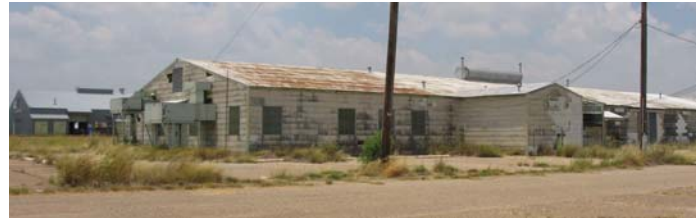
Formerly Used Military Building
